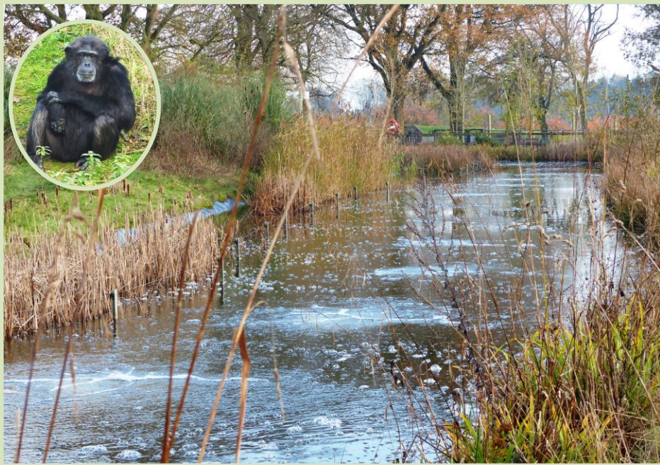
Left. Multiple diffusers used in a chimpanzee moat to help prevent ice formation. 30 diffusers used for a total power output of only 0.9kw.
